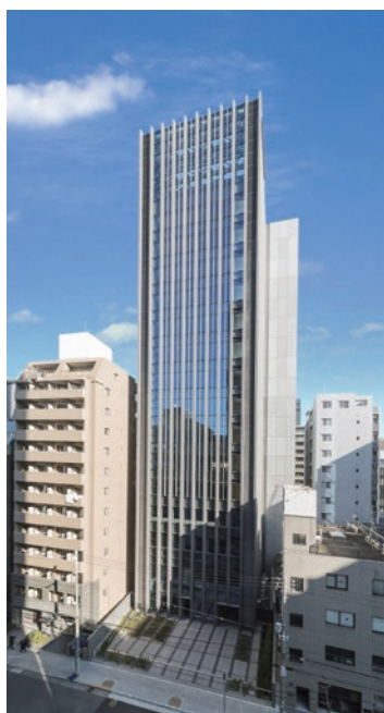
Promoted energy-saving initiatives, including switching to LED lighting at each workplace
