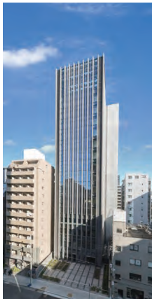
Promoted energy-saving initiatives, including switching to LED lighting at each workplace
